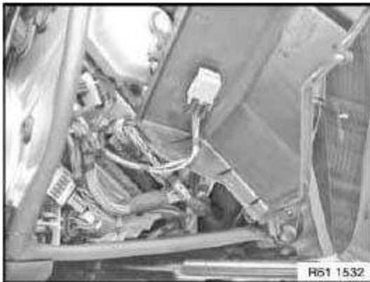
Fig. 207: Identifying Relay Courtesy of BMW OF NORTH AMERICA, INC.
